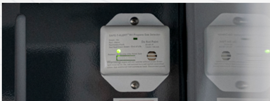
Fig 7.1 Propane gas detector
